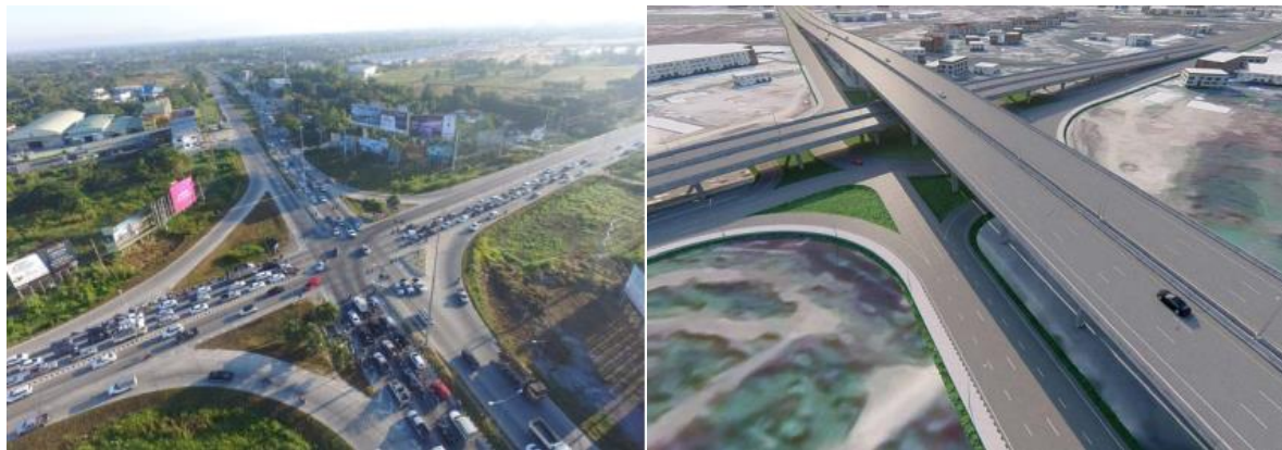
(a) Existing (Signalized)
