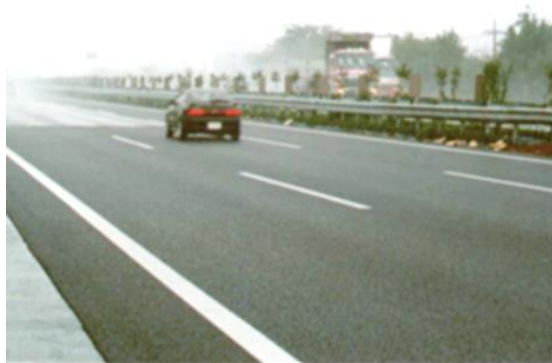
Figure 1 Visibility of porous asphalt on a rainy day.
