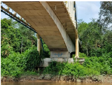
(a) Sub-structure condition of bridge
